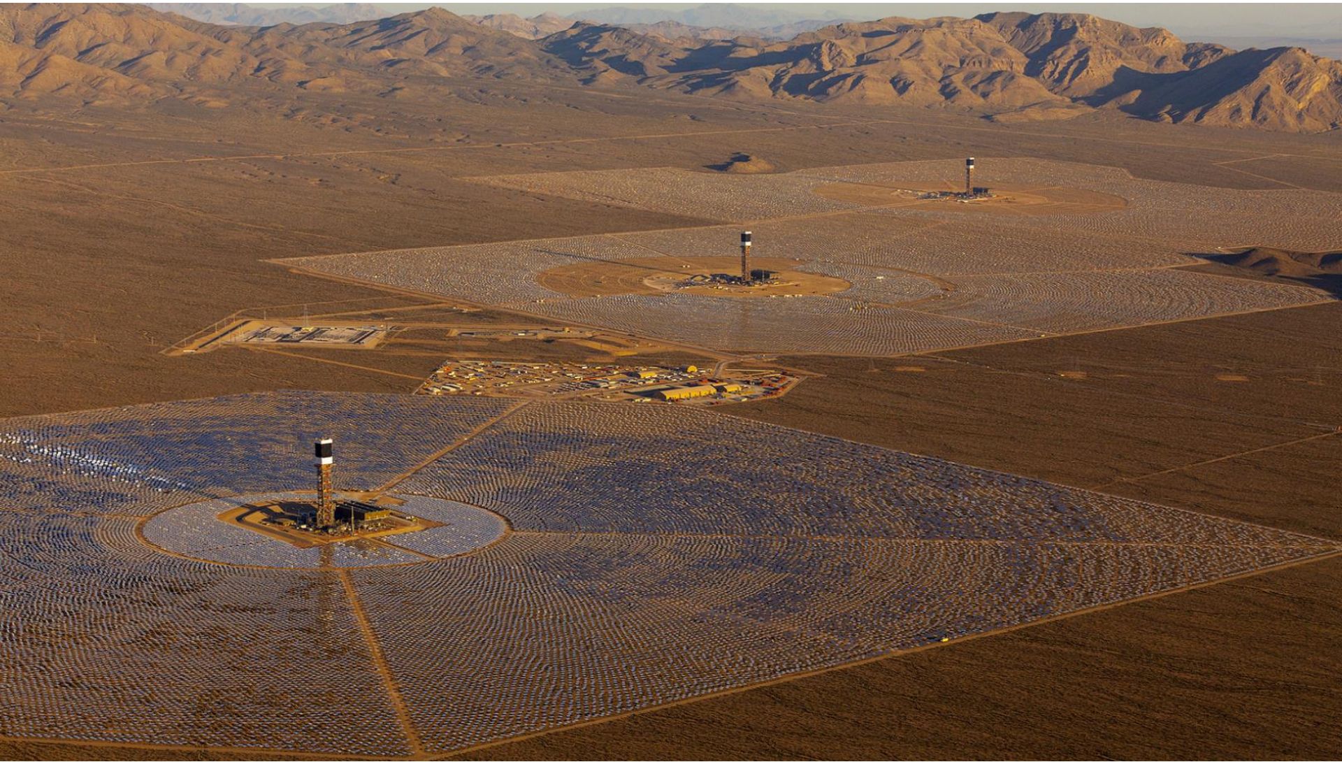
Ivanpah Solar Thermal Project 370MW San Bernardino County, CA
