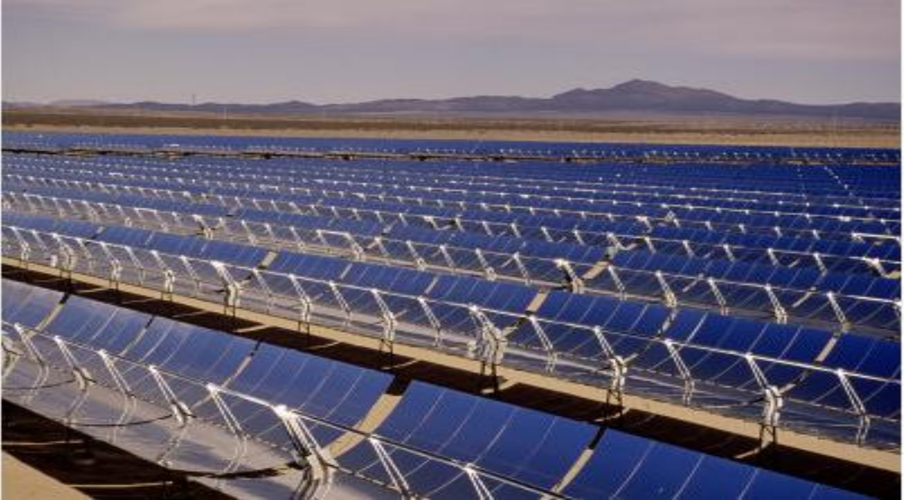
Solar Energy Generating System (SEGS) 310 MW San Bernadino County, CA
